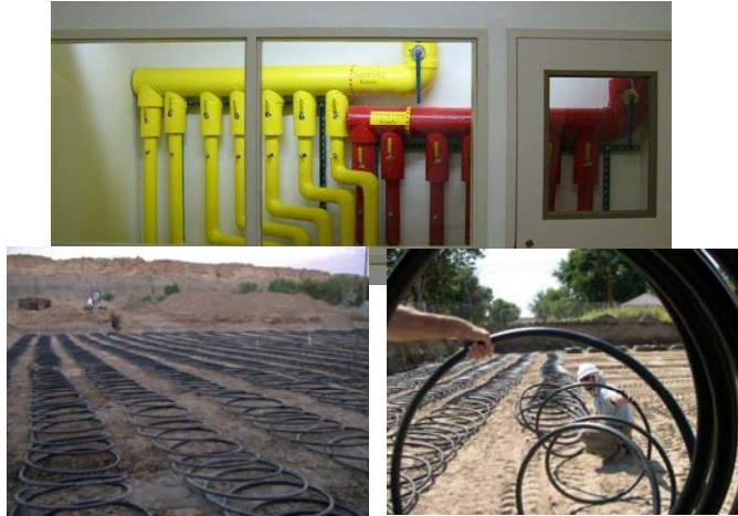
Greybull Elementary – Mechanical room under glass, LEED silver
