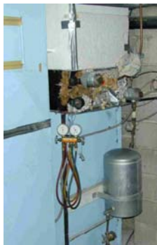
Air coil in old oil furnace
