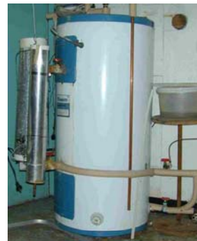
Desuperheater added to hot water tank
